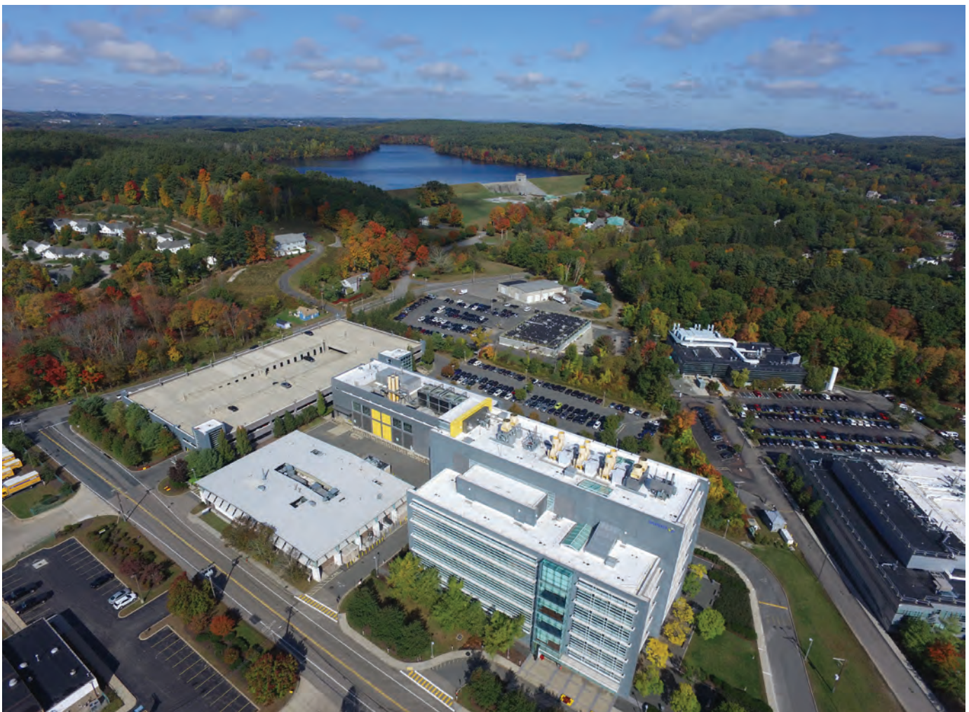
This 200-acre Framingham site includes Bose and Sanofi facilities.
